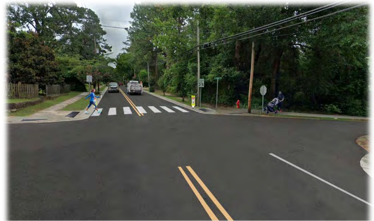
Crosswalk across Poplar Street connecting existing sidewalks on Elm Street to proposed sidewalks on Elm Street from Poplar Street to Sycamore Street.
